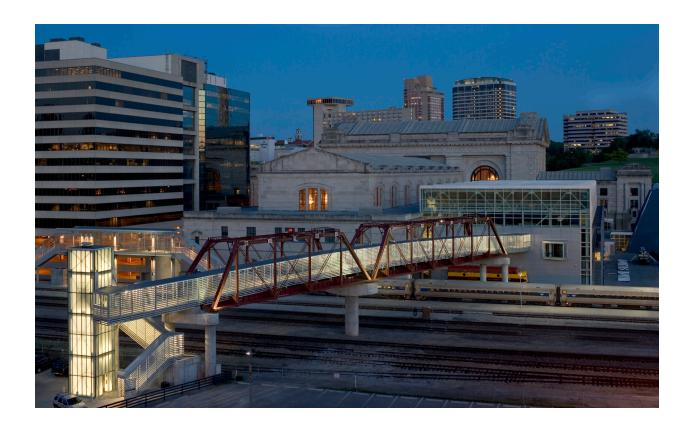
Once located at the riverfront in Kansas City, MO, the 250 foot long Pencoyd Railroad Bridge was built in 1892 and closed in 1970. BNIM worked to relocate the historic bridge to a new home in Kansas City's Freight House District, where it serves as a pedestrian link spanning the railroad artery that separates the Freight House and Crossroads Art Districts from popular civic destinations to the south including Union Station, Crown Center Plaza and Liberty Memorial.
